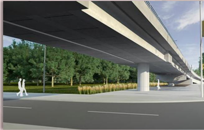
Elevated Guideway - $123M/mile
